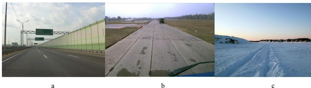
Figure 1. Types of lines on a road: (a) paint markings, (b) construction elements edges, (c) wheel tracks.
